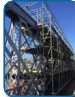
The project involved the provision of the access scaffolding and full containment to the underside and full length of the bridge in two separate phases, with strict time constraints a feature of the contract. Once the access was in place, SCA's coating specialists washed and blasted the steel surfaces to prepare them for the application of the new coat of paint.
