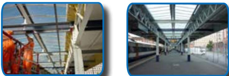
All coats of specified paint were applied to the riveted steel panels under controlled atmospheric conditions to ensure the covering was applied in line with the manufacturer's guidelines, and to the satisfaction of the main contractor, and Network Rail legislation.
